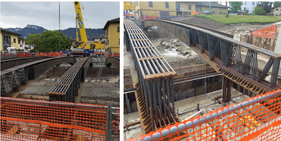
The new bridge with a single span of 25.6 metres and an 11-metre-wide section
