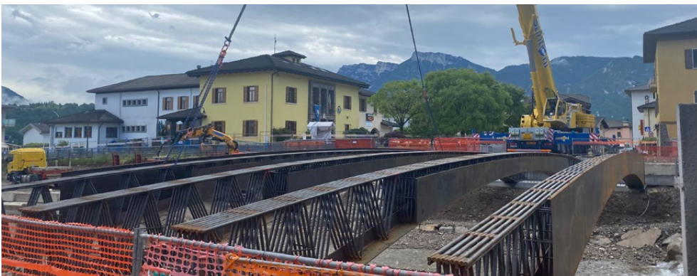
NPS beams for the new bridge in Calceranica
