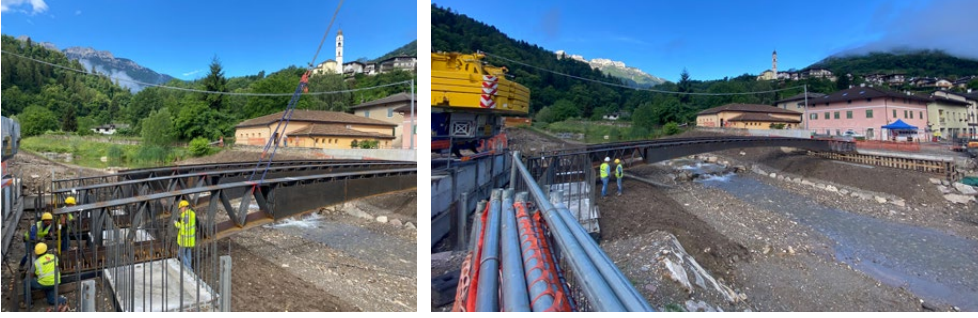
Construction of single span bridge, Calceranica (TN)
